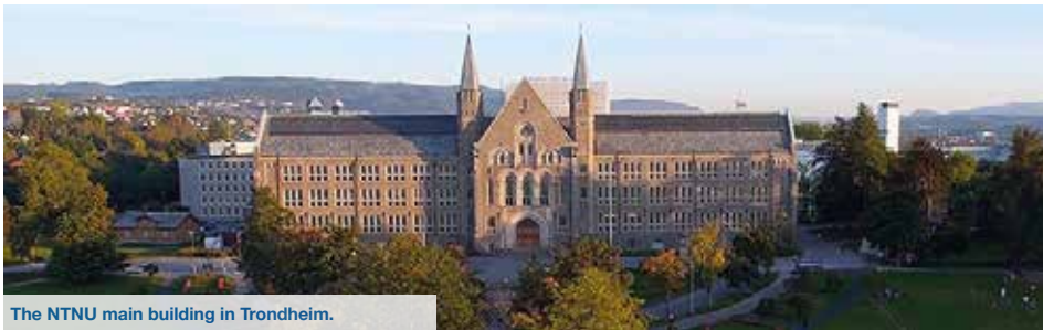
The NTNU main building in Trondheim.
